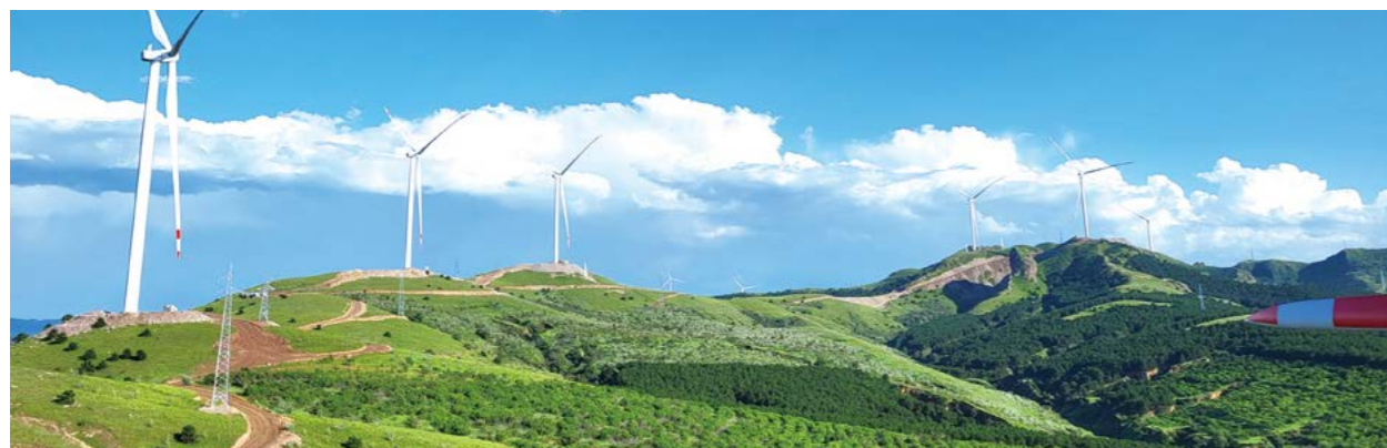
GCL-ET Liaoning Juxin 50 MW Wind Power Project
