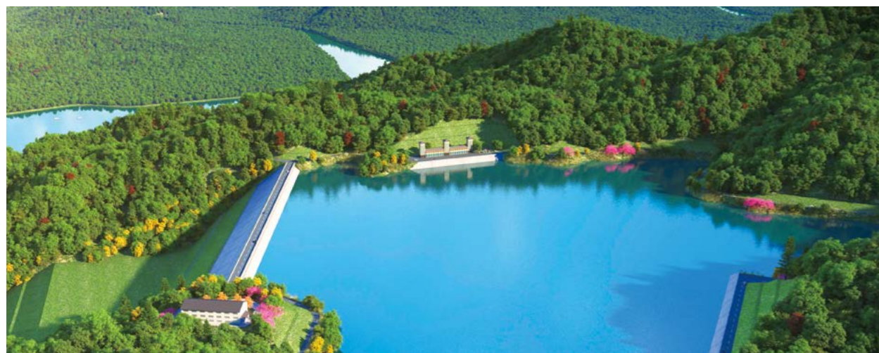
Aerial view of GCL Zhejiang Jiande Pumped Storage Power Station
