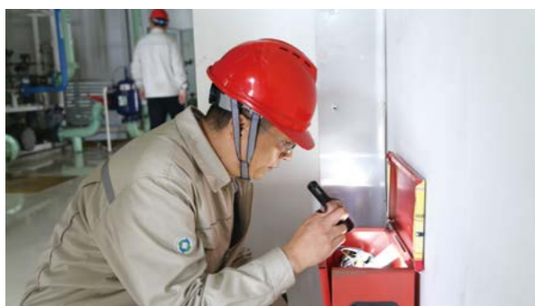
"Fire Protection Awareness Month" campaign: Wuxi Blue Sky carried out a fire protection inspection based on the fire prevention characteristics of autumn and winter
