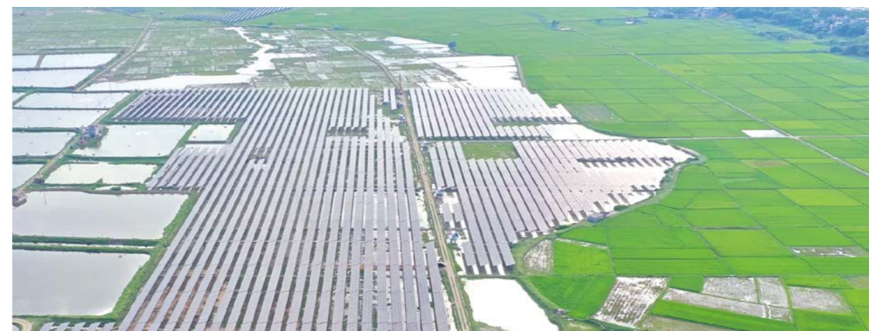
Guangxi Qinzhou Farmland PV System Project
